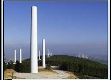
Fig 8(a) Tubular tower
